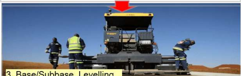
3. Base/Subbase Levelling
