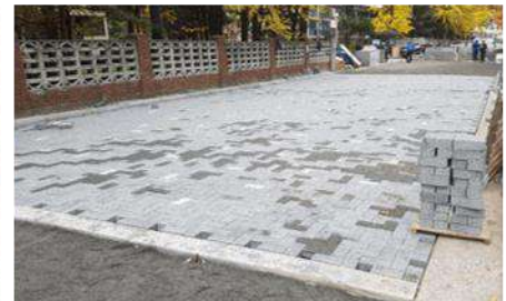
Block Paving on Permeable Road
