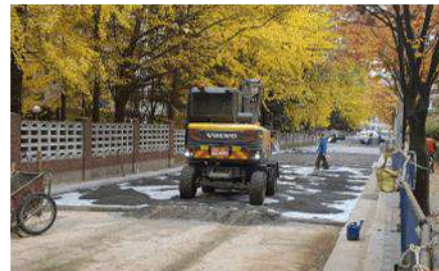
Block Paving on Permeable Road
